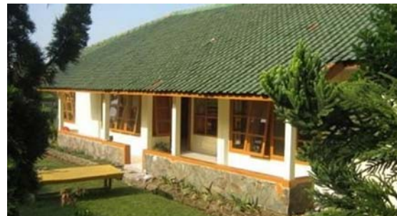
One of the renovated children's dormitories
